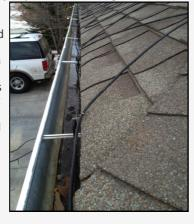
2. Next, have heat wires installed on roofing shingles and in gutters and downspouts on
